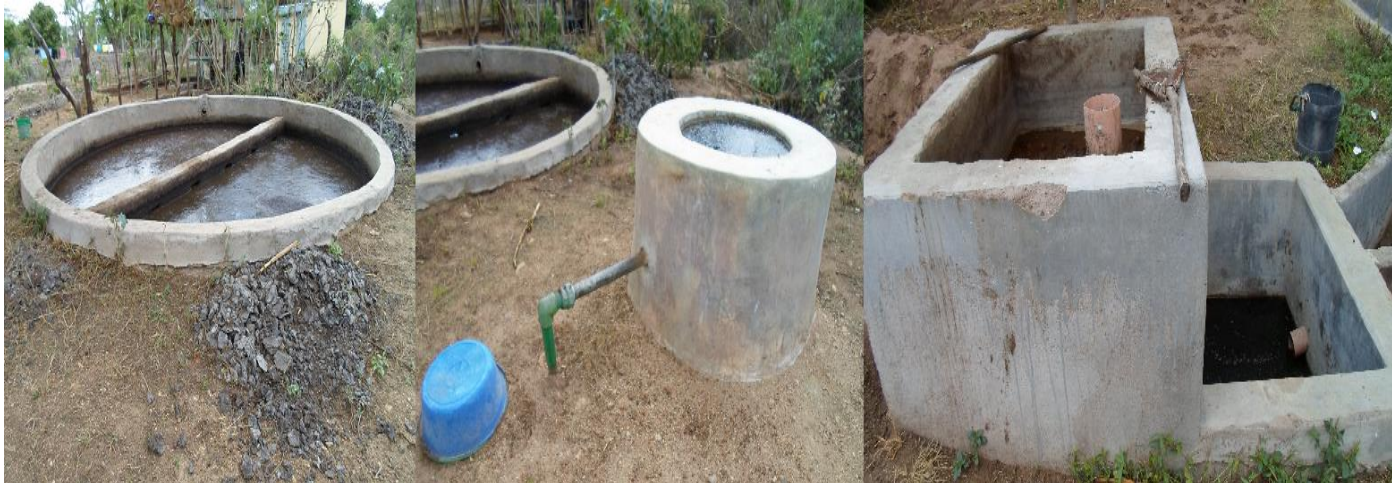
Figure 3.4 Biogas facility at Katulani SS. Output chamber is shown to the left, biogas output in the middle and slurry input with mixing device to the right
